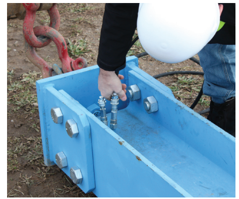
Step 3. Verify the connections of supplied 6' (1.8m) hoses are secure. Note, opposite end of hoses have 1/2" male NPT fittings.
