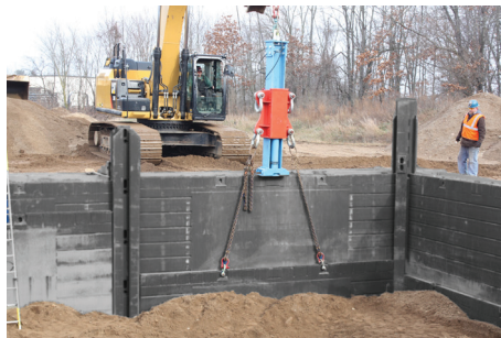
Step 8. Using power pack or auxiliary system, begin process of applying force to remove panel.
