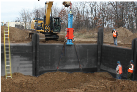
Step 7. Have crew connect distributor supplied rigging to desired panel.
