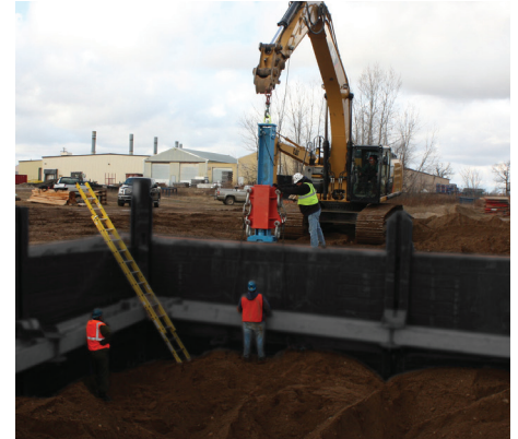
Step 6. Bring Panel Puller system to Slide Rail System, setting Panel Puller on a stable area.
