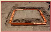
Assemble initial ram and extensions. If using multiple levels of rams, assemble the rams and extensions and stack on top.\*
