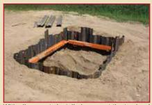
With all supports installed, connect the top level of the Pro-Brace to the bracing supports with Hanging Chains and pressurize system.
