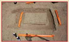
Dig initial pilot cut (2-3') and stage one leg of the Pro-Brace Hydraulic Rams. If using multiple levels of rams, they may be stacked upon each other to speed up installation time.\*
