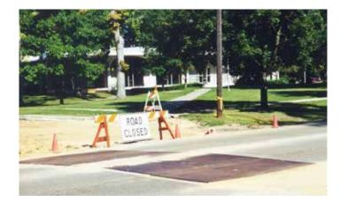
Trench widths are based on an analysis per the 14th edition of the "standard specification for highway bridges" by A.A.S.H.T.O. An assumed axle loading of 12 tons with a 30% impact factor was used. The axle length is 6 feet; therefore the number of wheels carried by a plate depends on the roadway width.
